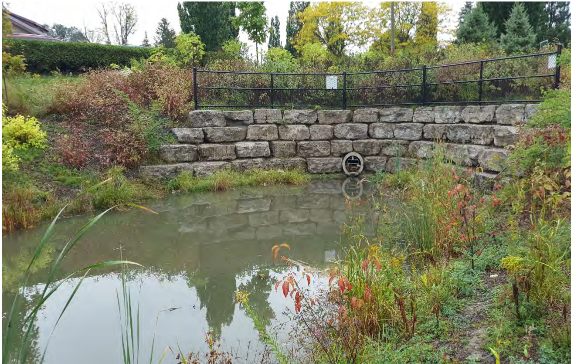
Photo 6 - Inlet #2 forebay looking west.
