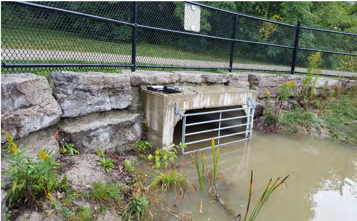
Photo 1 - Inlet #1 facing north.
