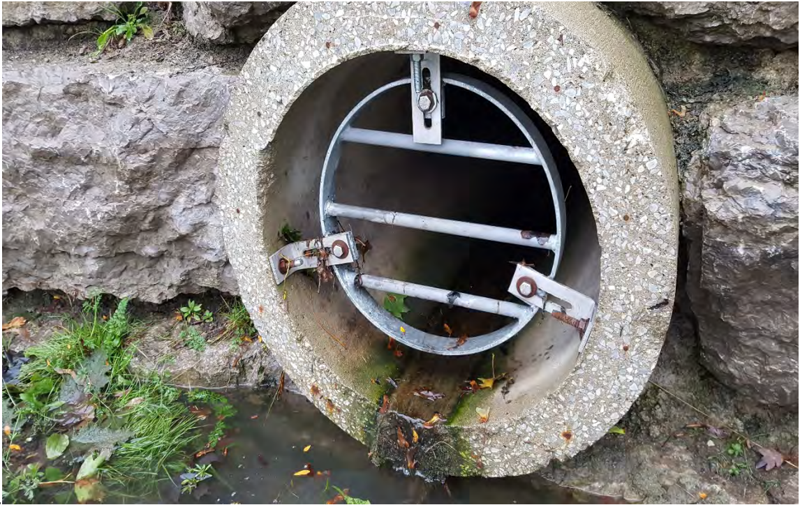
Photo 9 - Debris removed from inlet #2 culvert.
