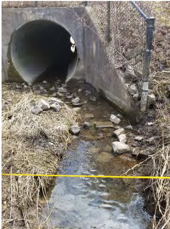
Photo 5 - SCH1 Upstream Culvert (03/29/2019)
