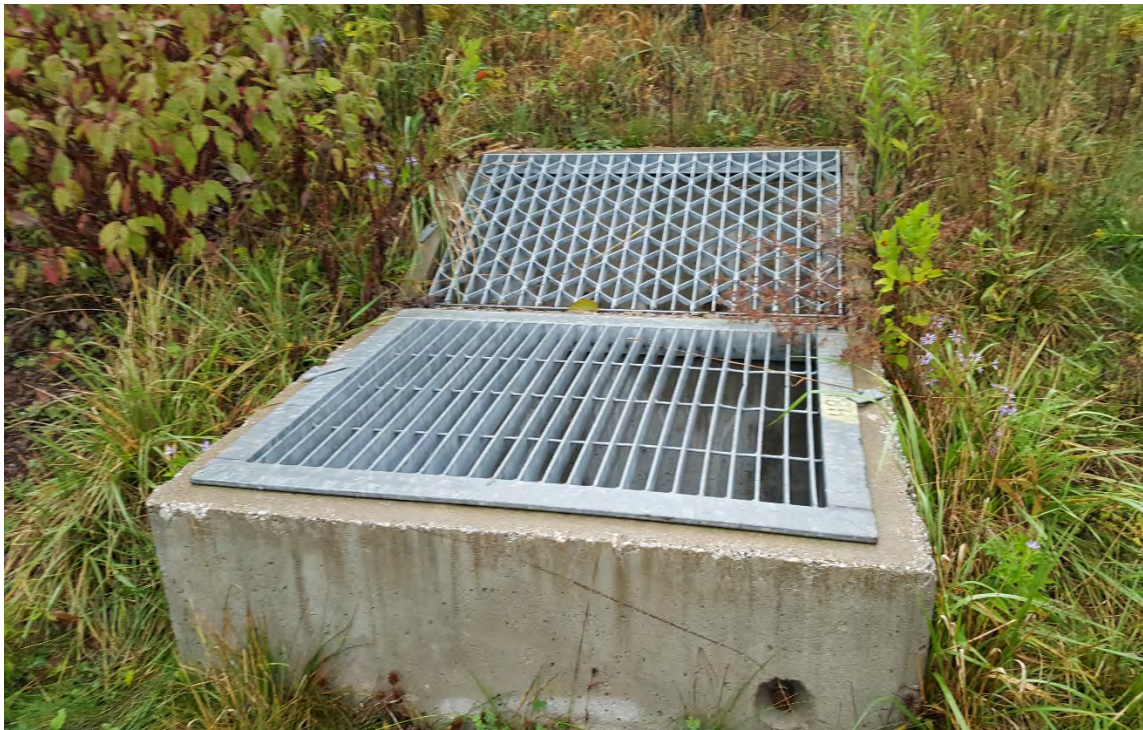
Photo 53 - Pond outfall grate structure.
