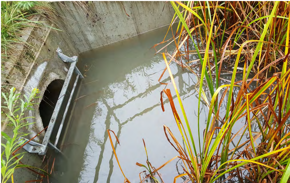
Photo 16 - Outfall culvert and sampling location.
